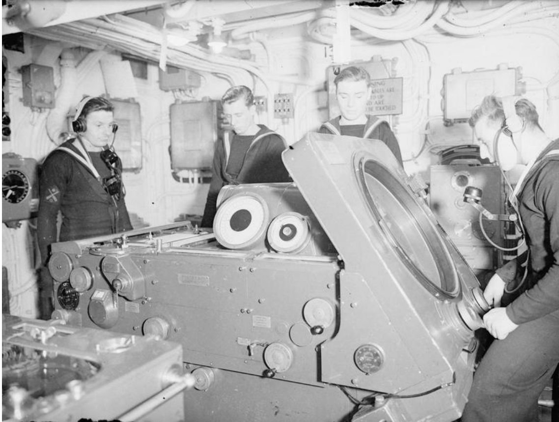
RN High Angle Control System Fire Control Computer (1930s/40s)
